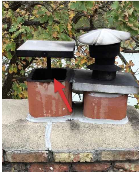
Top Sealing Chimney Damper
