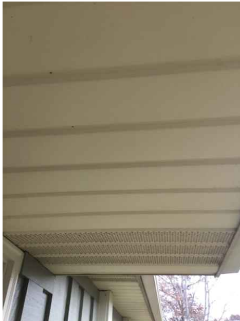
Over front entry way
