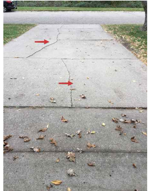
View from garage looking at street
