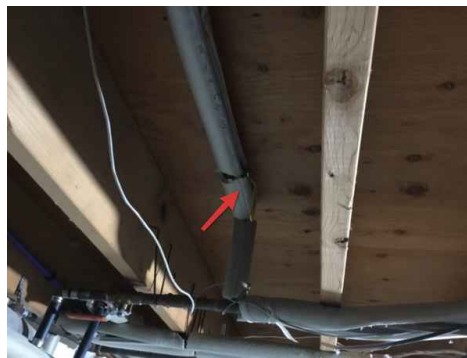
Shut off valve - Back hose bib
